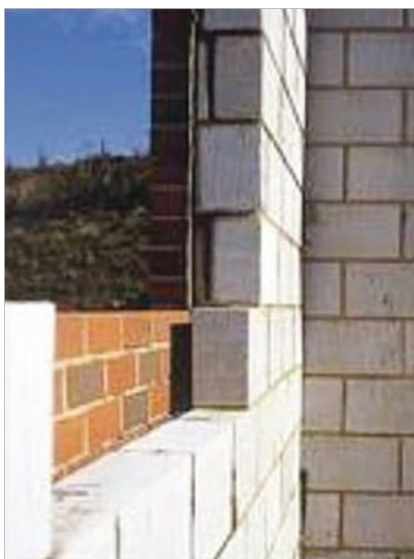
Modern cavity walls under construction.
